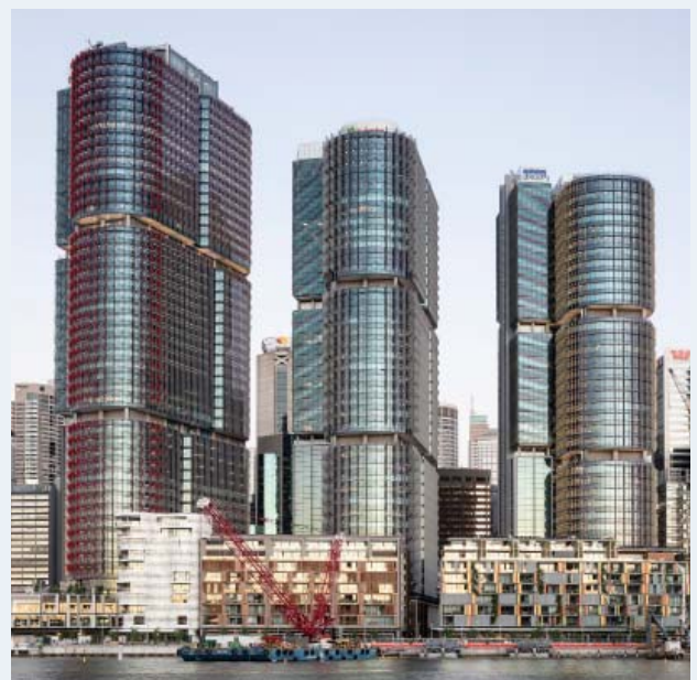
Barangaroo South Precinct / Source: Lendlease
